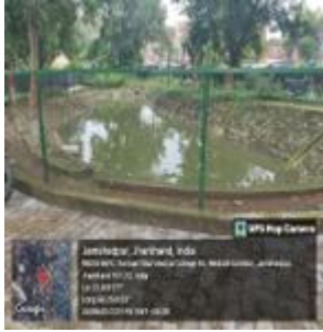
Construction of tanks & Bunds
