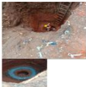
Bore well /open well recharge
