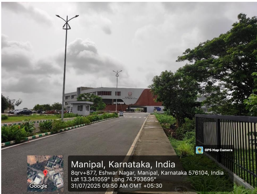
Street light and foot path
